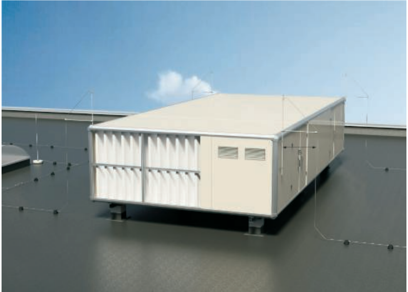
Insulated intercepting device with separating spacing (s)
