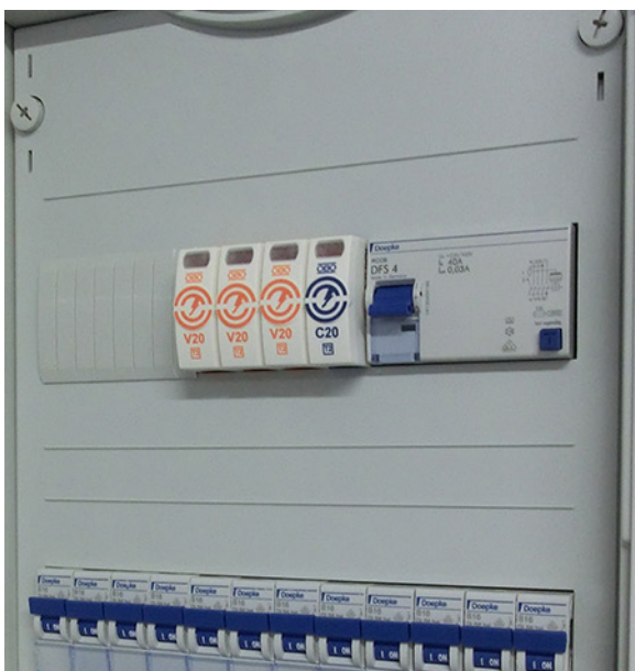
Image 2: Surge protection type 2 in the control cabinet, V20 3+NPE-280
