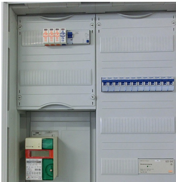
Image 1: Combination arrester type 1+2 in the main distributor, V50 3+NPE-280
