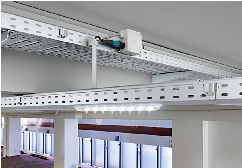
Image 3: Surge protection type 2 in the junction box, mounted on the cable support system, ÜSM-LED 230
